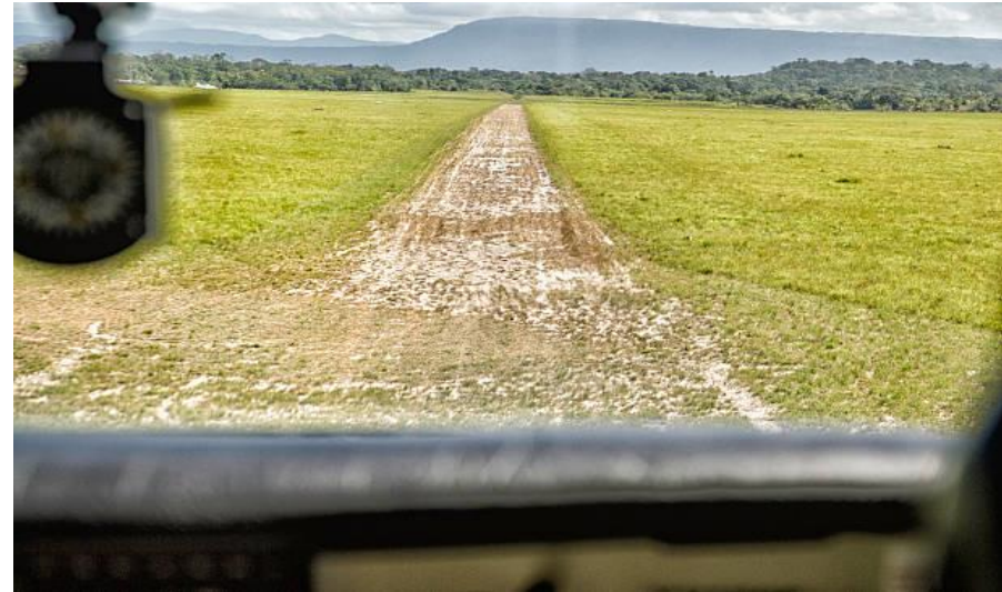
There are at least four drainage ditches crossing this airfield, how many can you see from this low angle? An intermediate pass first would have been better.
