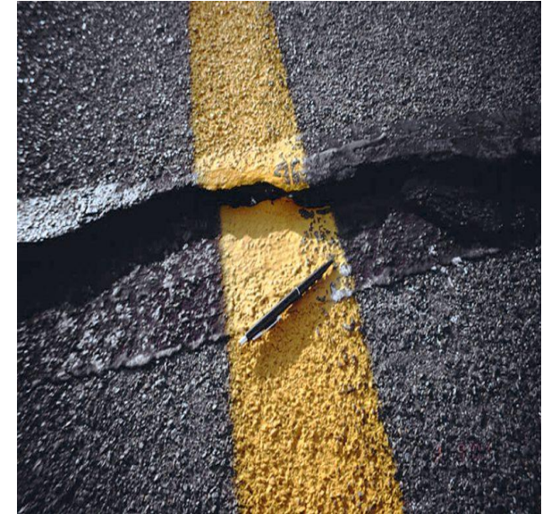
Could you see this serious runway crack from pattern altitude? A low level pass would be better.
